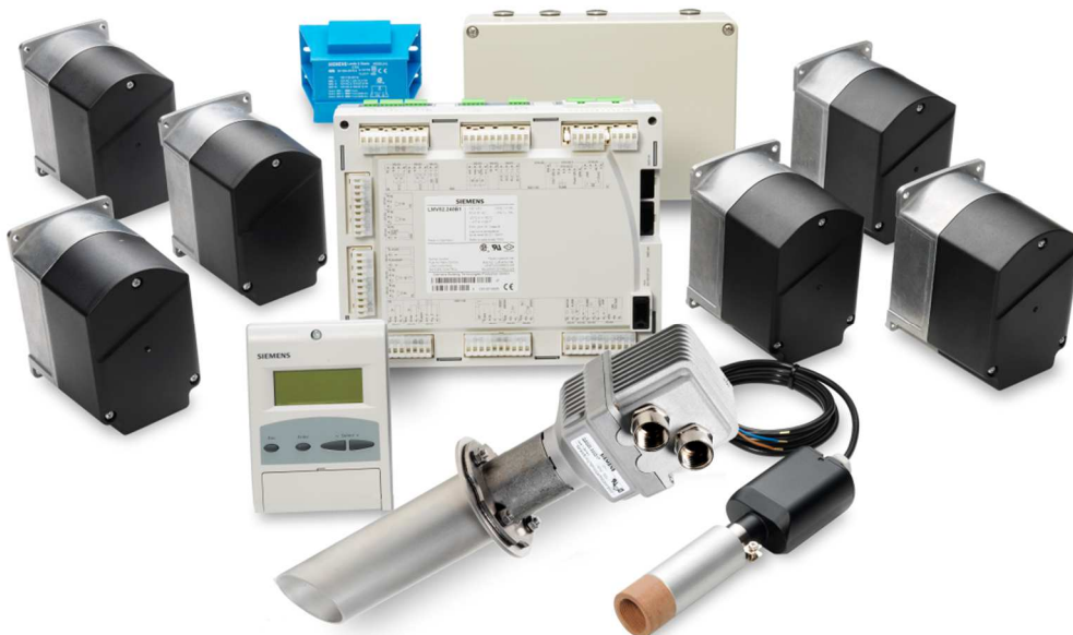
Figure 1-1.1: The Main Components of an LMV5 System
