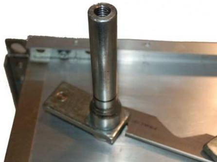
**Figure 3: Tapped Hole in Shaft Extension**
